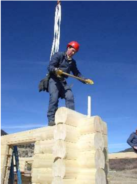
Diving a wooden peg with the 8lb sledge
